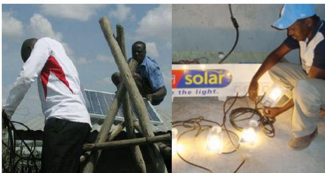
The installation of a solar panel on the roof of Mr Moite's shop roof and a typical battery and inverter pack powering light bulbs
