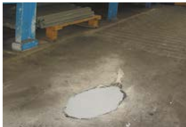
Renovation of flooring in a rolling mill
