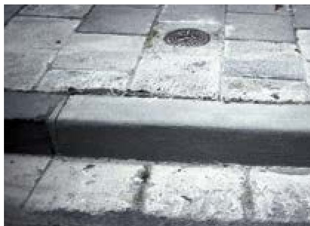
Renovation of kerbstones with SILIKAL® R 17 mortar
