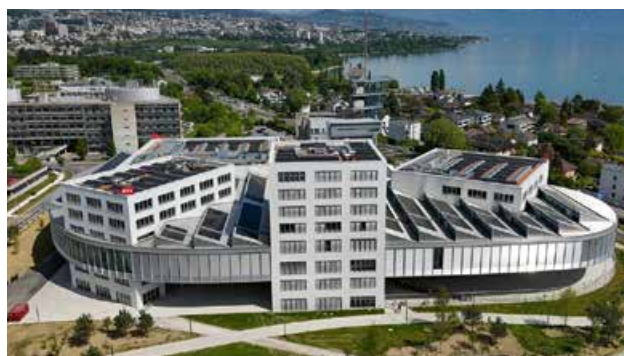
Le nouveau site RTS Lausanne-Écublens. © RTS/Jay Louvion
