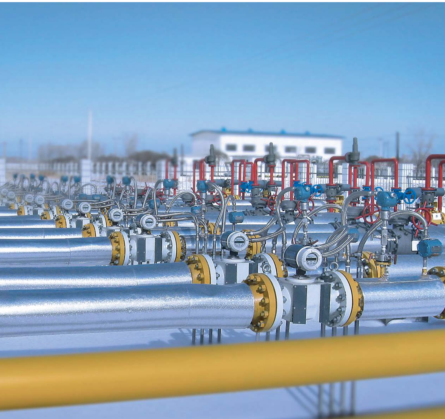
Natural gas pipeline in Bawu-Changnan using FLOWSIC600
