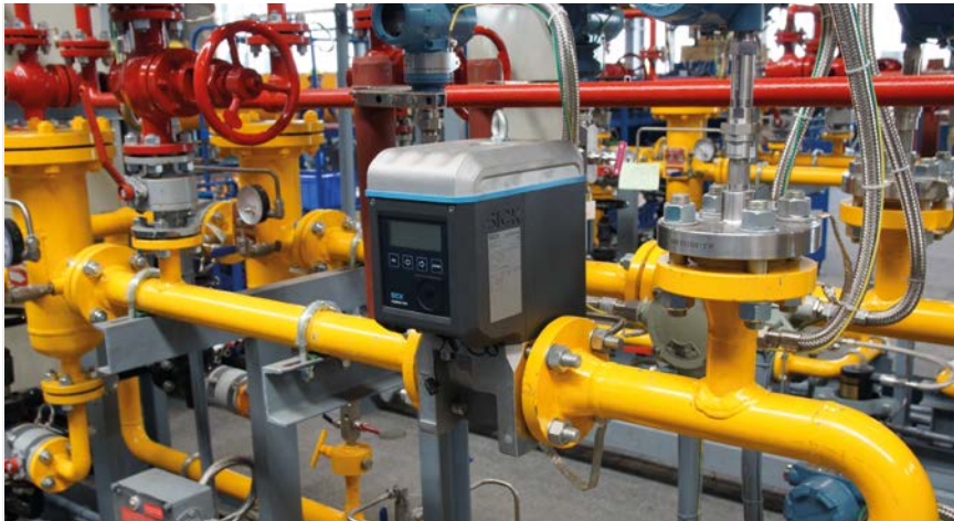
FLOW5IC500 installation
